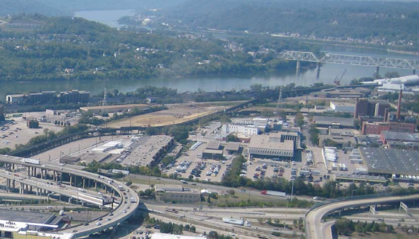
Energy development plant in Cincinnati, US
